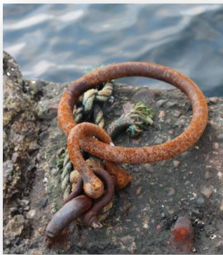
Ulva Ferry Pier Photo: Alasdair Satchel
